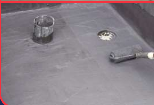
▶ Applying CW Seal 900 on the wall and floor to avoid the water from seeping in the structure.
